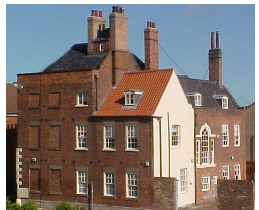
Fig.13 Blaydes House, High Street
